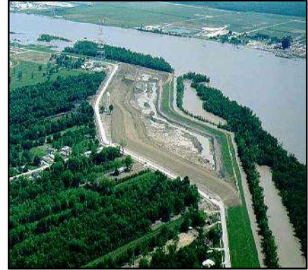
Photo 2. Setback levee (photo courtesy of MVN-USACE).
