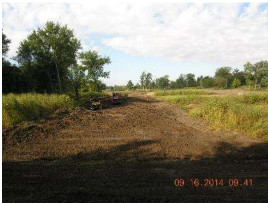
Photo 11. Berm modifications (photo courtesy of MVS-USACE).
