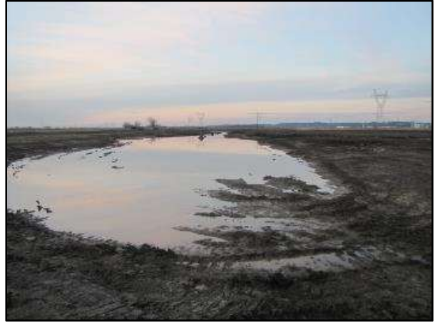
Photo 16. Wetland excavation (photo courtesy of MVS-USACE).
