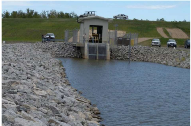
Photo 18. Pump station (photo courtesy of MVR-USACE).
