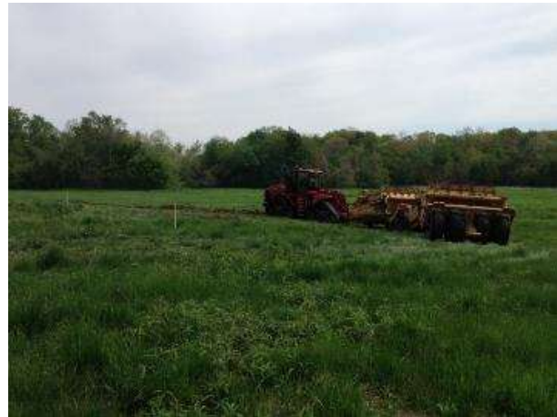
Photo 14. Channel excavation (photo courtesy of MVS-USACE).
